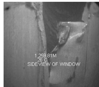
The ViewMax provides an excellent assessment of the damage to the lower edge of a window in this multilateral completion
