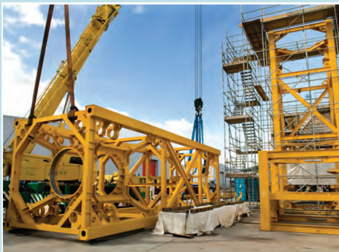
Winch frame arrives at Hydrakit
