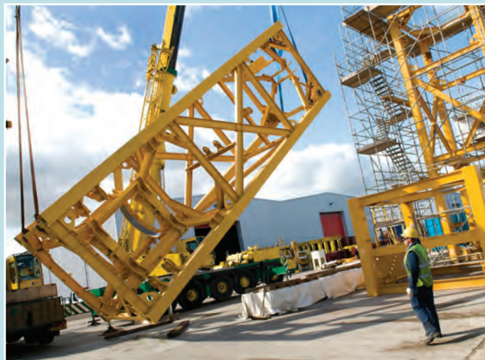
Winch frame is upended using two cranes
