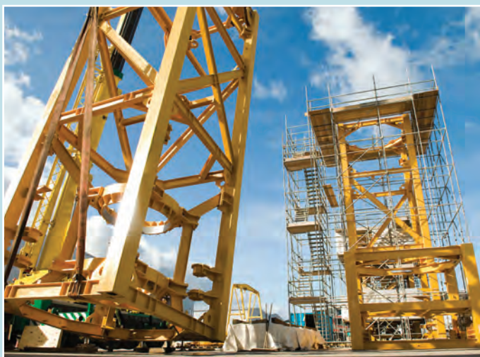
Winch frame is upended to the correct position
