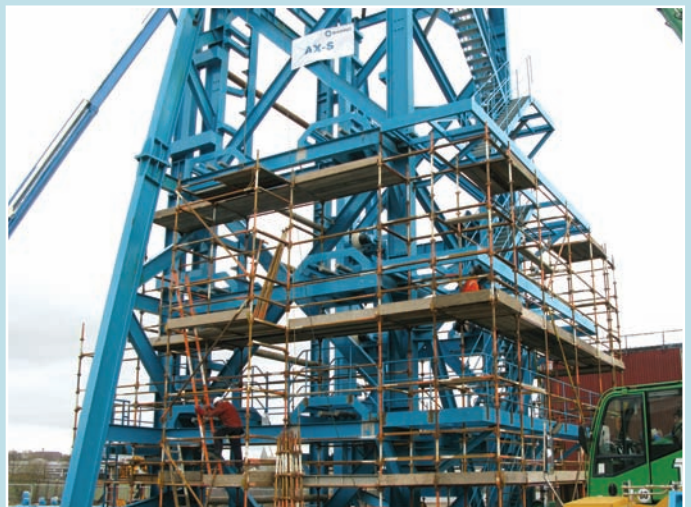
The handling tower assembly at King George V dock in Glasgow
