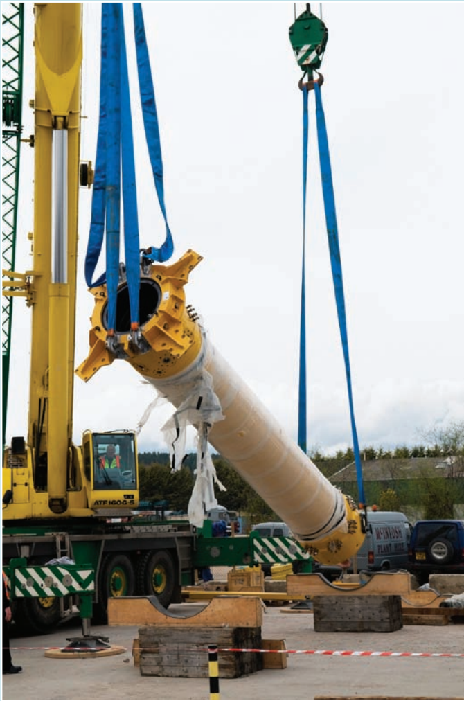
TSP pressure housing being moved into the vertical position
