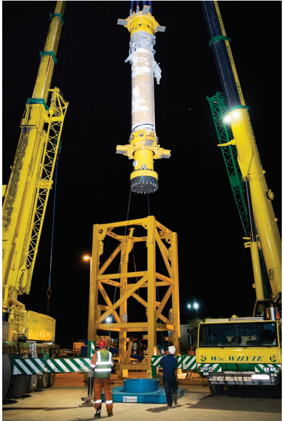
Main pressure housing being lowered into TSP frame
